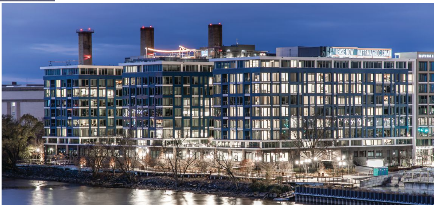
TSI Corps installed window wall and stick-built curtainwall for the 1900 Half St. residential project in Washington, D.C., designed by Antunovich Associates.
